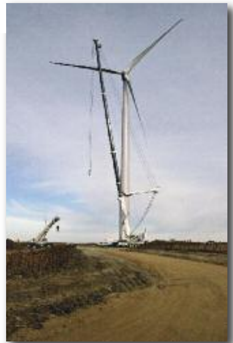
To help speed up construction in November, a special crane that uses a hydraulic boom was brought to the site of the wind farm.
