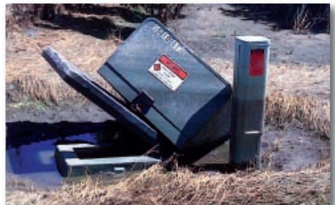
Above and below: Hundreds of meters and transformers like these were damaged in the flood.
