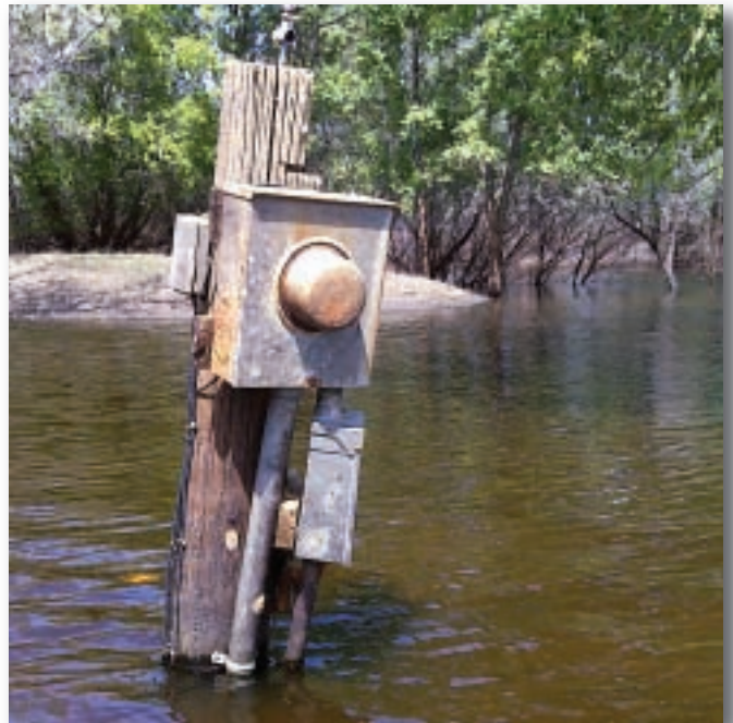
Above and below: Hundreds of meters and transformers like these were damaged in the flood.
