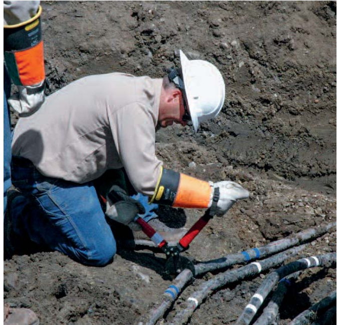
Verendrye lineworkers repair an underground power line after it was damaged by a backhoe. Hitting an underground power line can be dangerous and can also cause outages.
